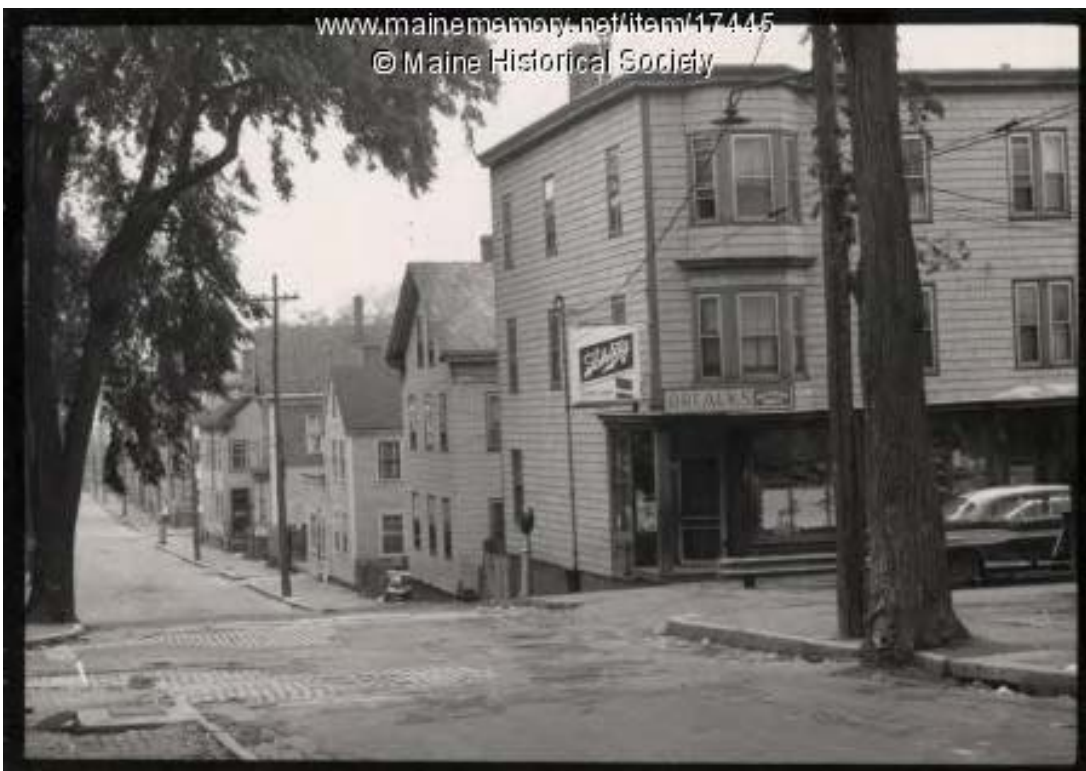
Portland's former Little Italy. These buildings were destroyed by Franklin Arterial. Photo courtesy of Maine Memory Network. Available from http://www.mainememory.net .
